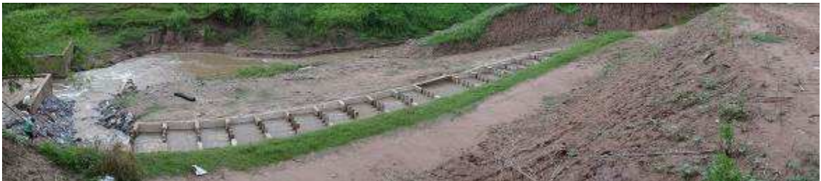
Figure 7. Panoramic view of the lower fishway channel section of the completed Pak Peung fishway.
